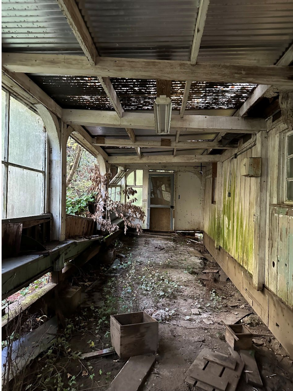
Photo 15: Cabin Interior – Enclosed Porch Facing South
