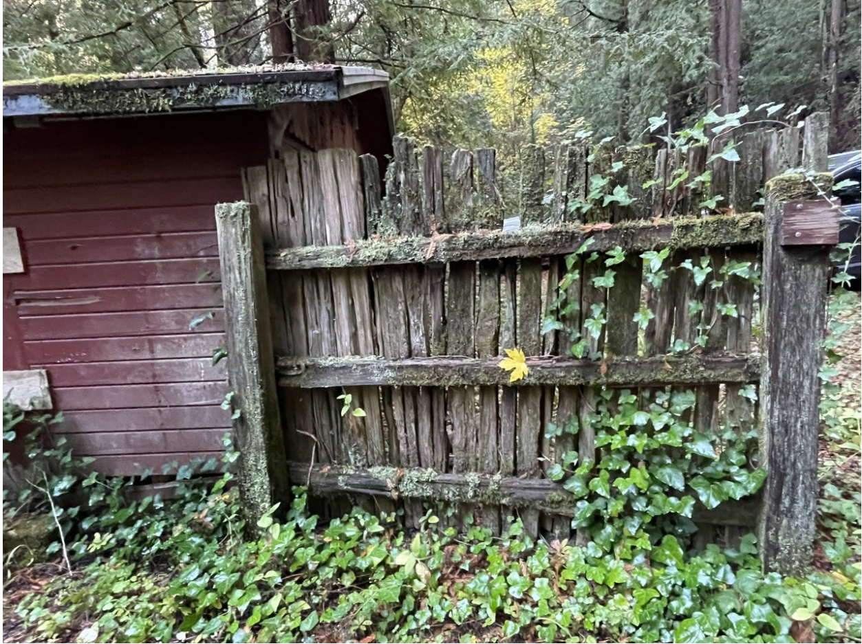
Photo 17: Cabin Site – Fence at Garage
