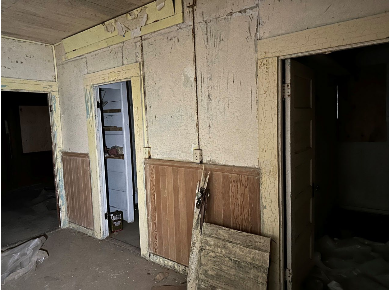
Photo 9: Cabin Interior – Kitchen North Wall
