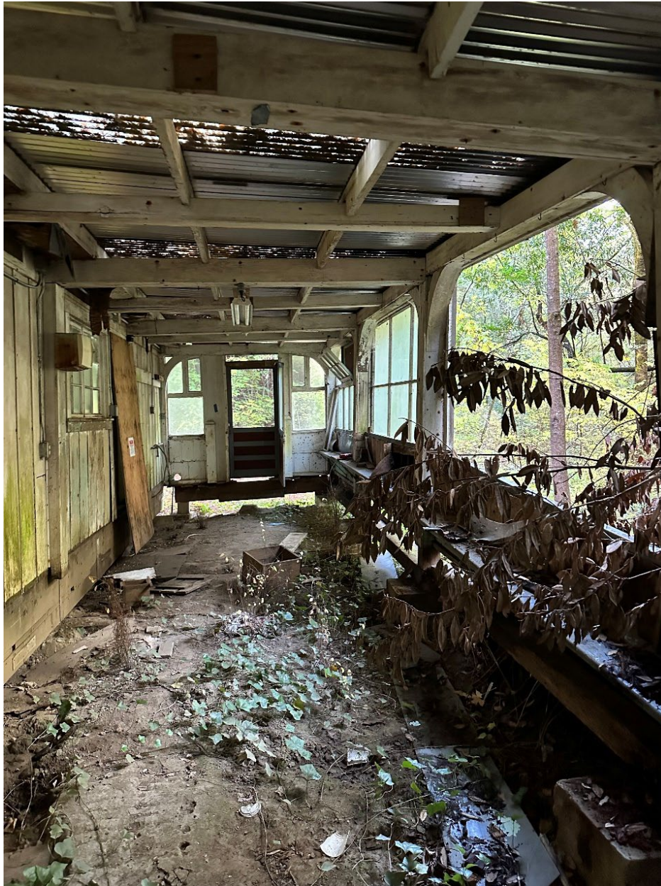
Photo 14: Cabin Interior – Enclosed Porch Facing North
