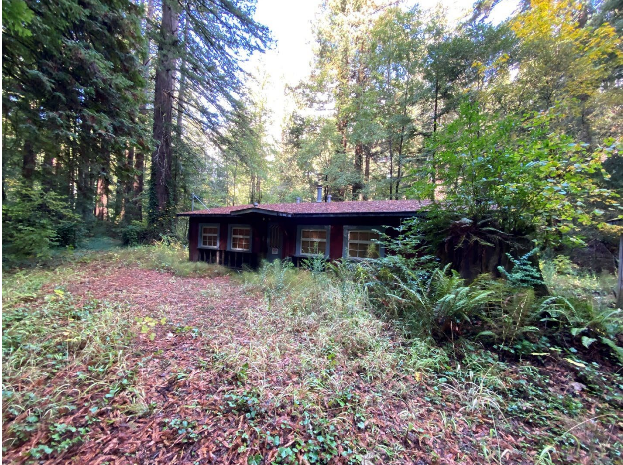
Photo 2: Cabin Exterior – West Elevation of Cabin with Redwood Stump
