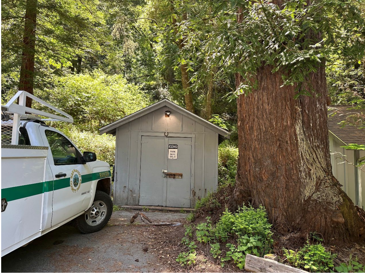
Photo 24: Sam McDonald County Park – Storage Shed at Park Headquarters
