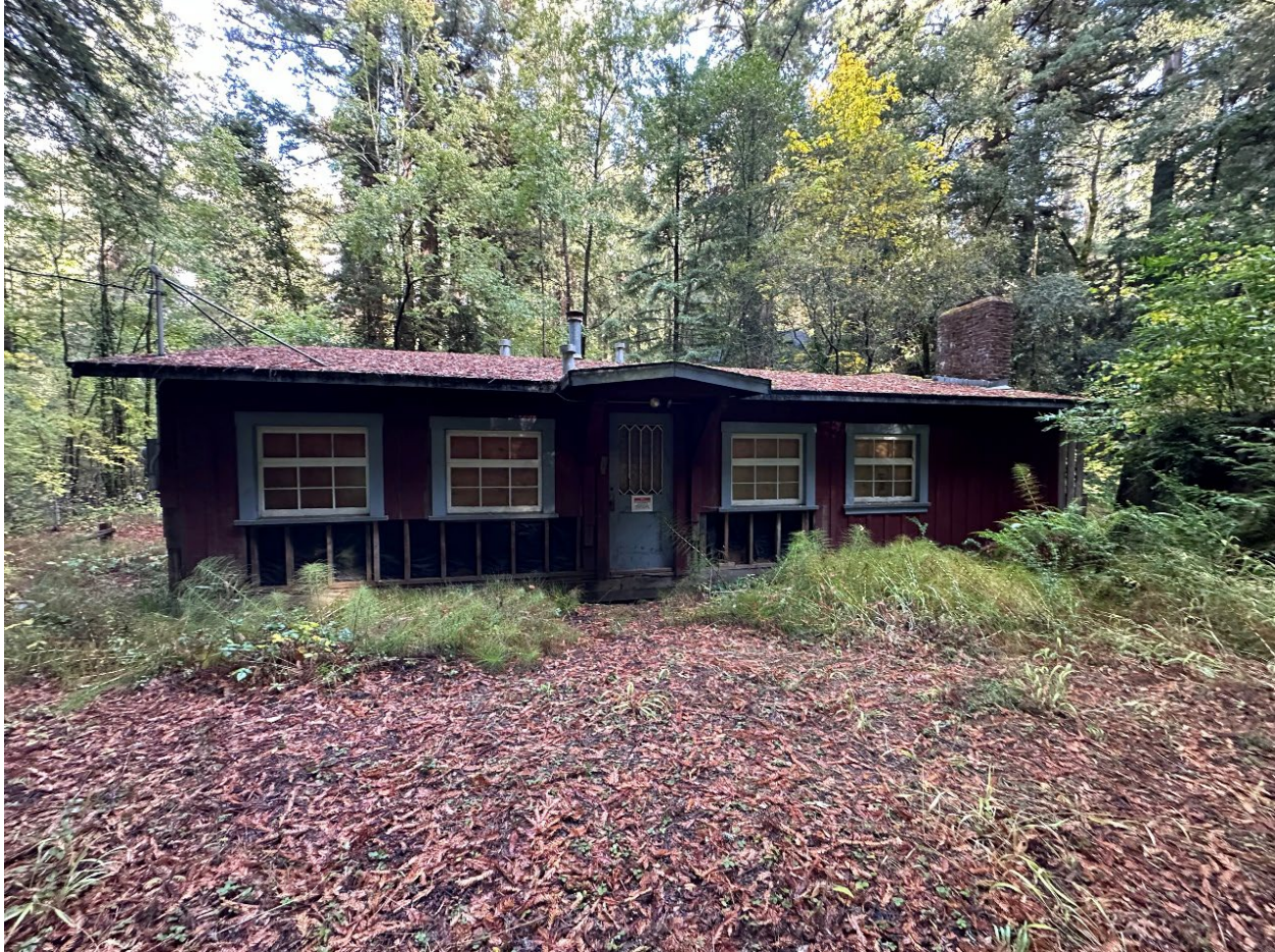
Photo 1: Cabin Exterior – West Elevation
