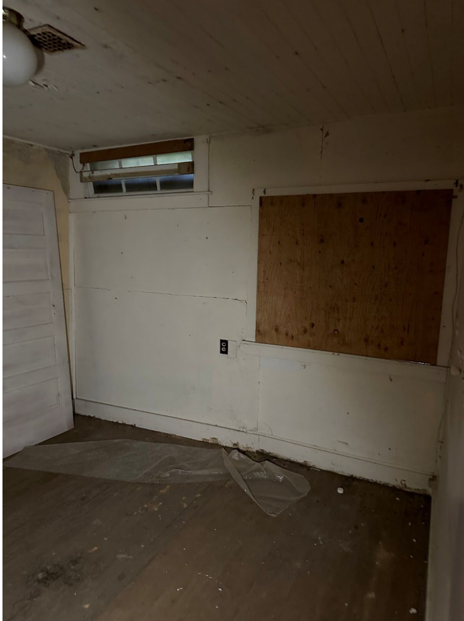
Photo 12: Cabin Interior – Bedroom Facing South
