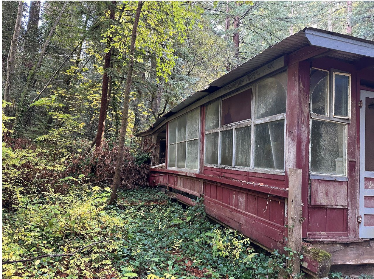
Photo 4: Cabin Exterior – East Elevation from Northeast Corner
