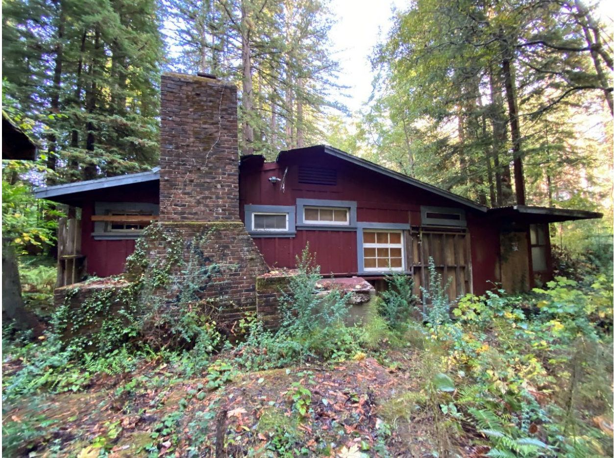
Photo 5: Cabin Exterior – South Elevation
