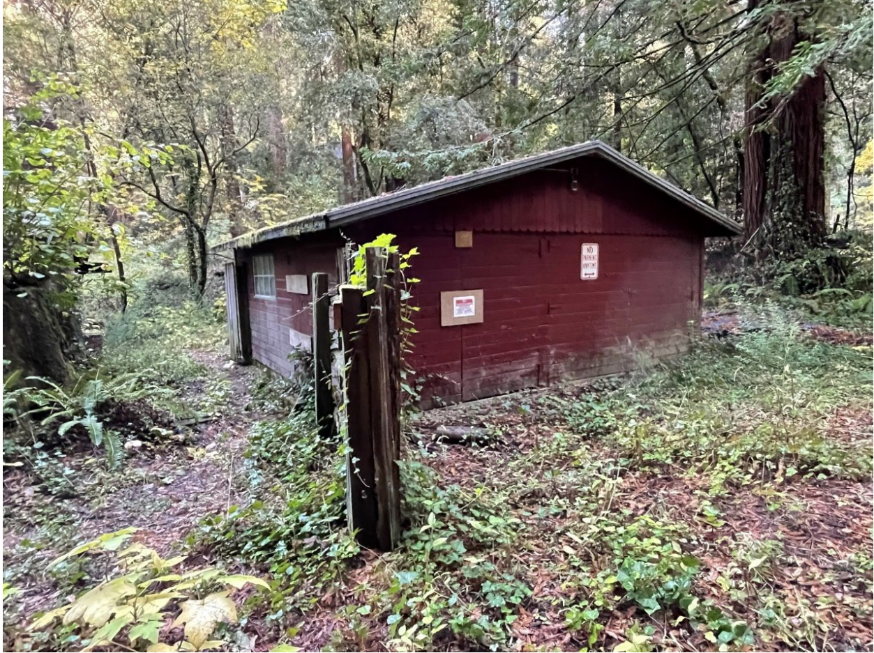
Photo 16: Cabin Site – West Elevation of Garage
