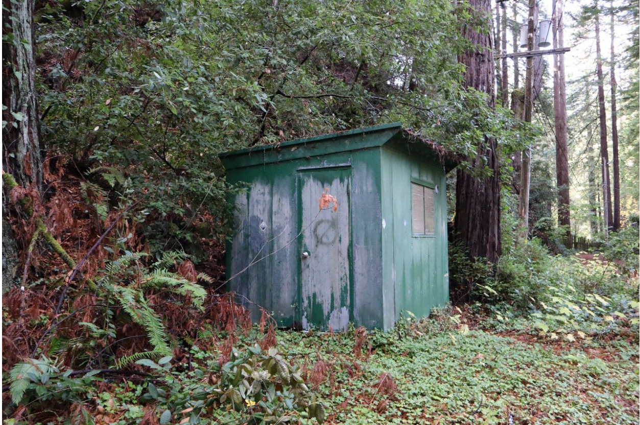
Photo 19: Cabin Site – Pump House
